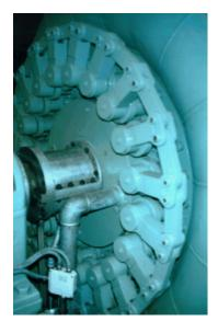
Photo 6.4: Horizontal axis Francis turbine guide vane operating device
