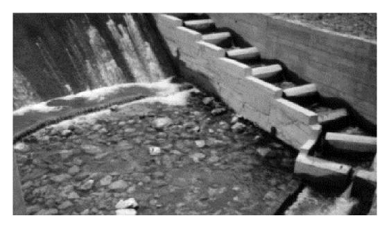
Photo 7.14: Fishpass with vertical slots
